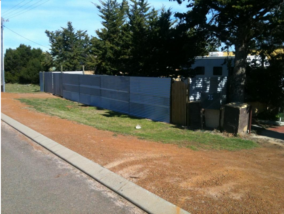
Subject Site and front fence
