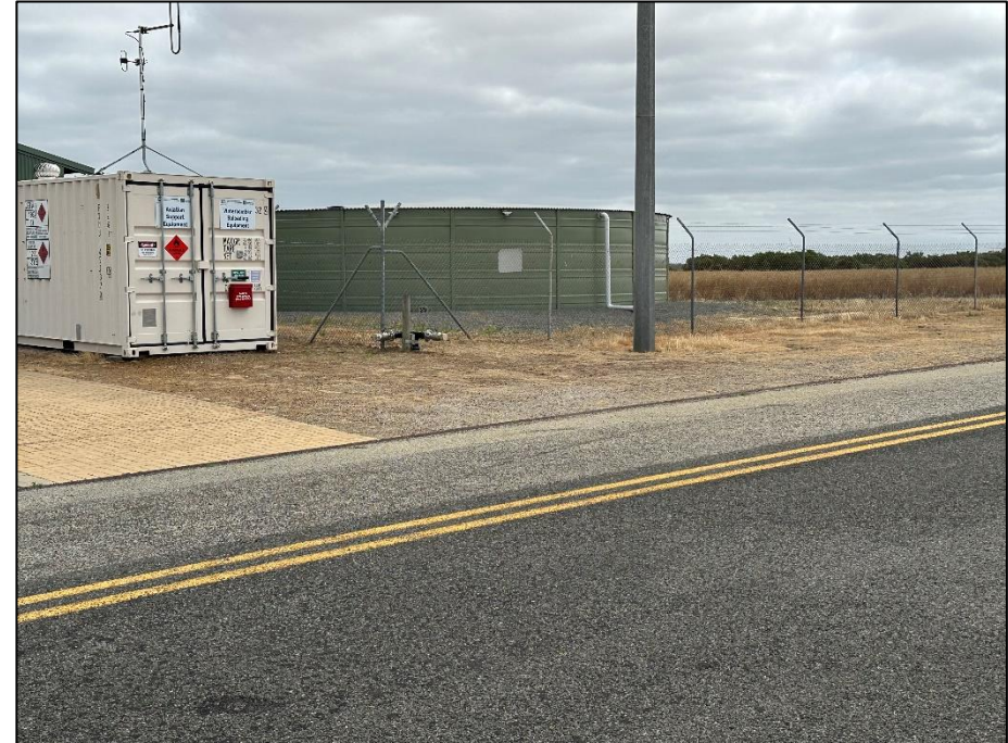
Figure 22 DBCA emergency firefighting facilities
