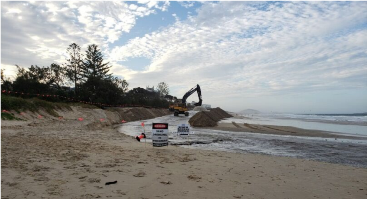
Figure 7-1 Beach nourishment underway at Sunshine Coast, QLD
