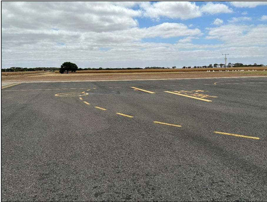
Figure 16 Gravel aircraft parking apron (east)
