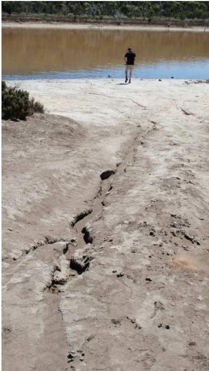
Phillips River Reserve - River bank erosion associated with boat launching site (Melanie Price, 2011).
